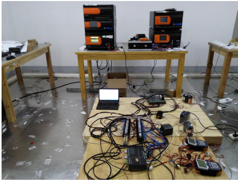
Photograph 23: Voltage Dips/Interrupts Test Configuration
